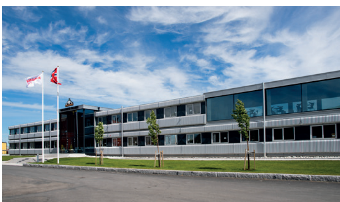
MASONITE MAIN OFFICE IN SWEDEN
